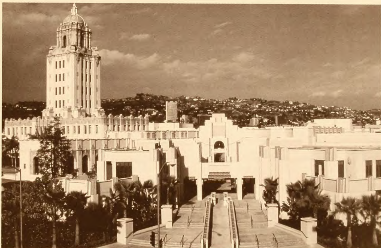
Charles Moore e The Urban Intervention Group, Beverly Hills Civic Center, Los Angeles, 1980. Viste. Foto T. Hursley. Pianta.
