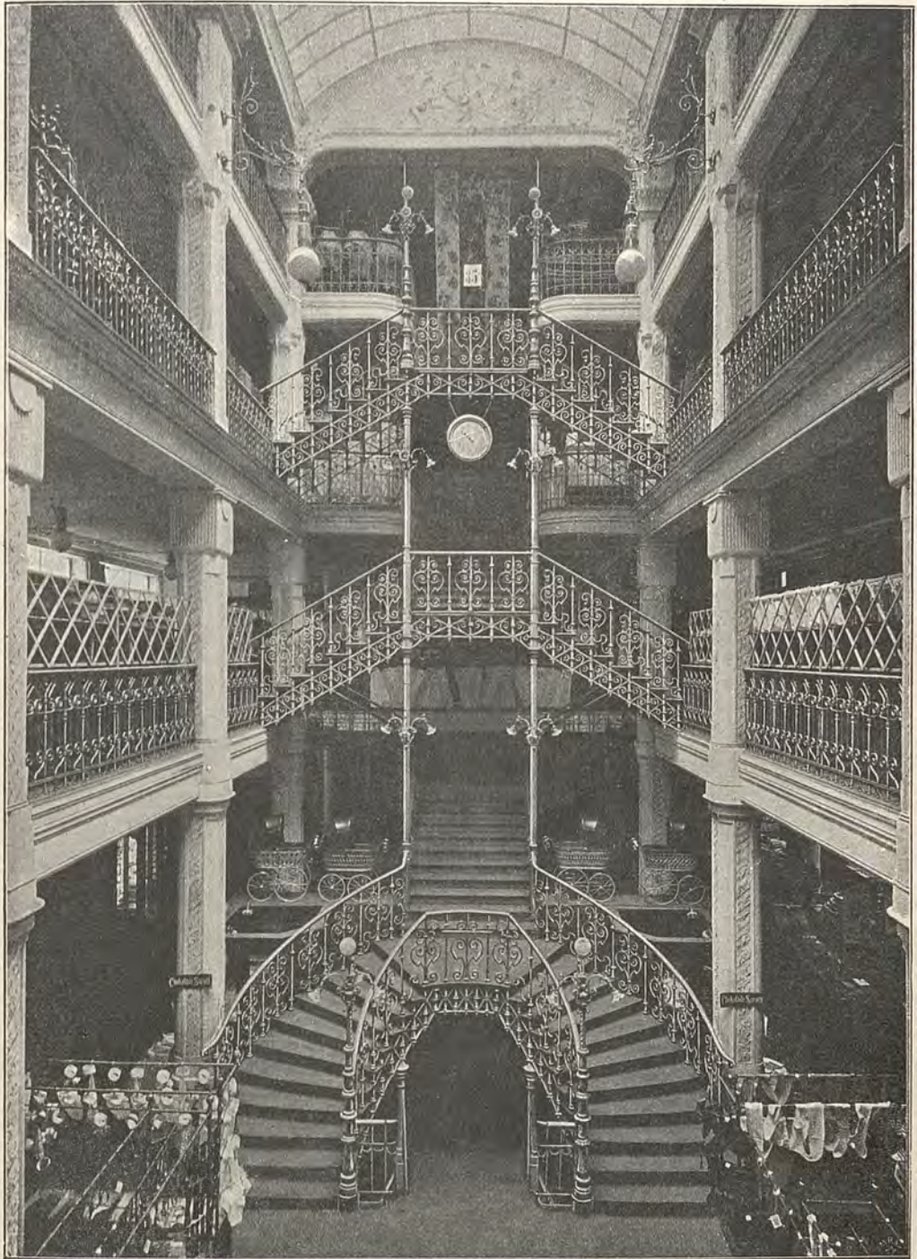
Scala metallica sistema Joly pei magazzini Wronker in Hannover (Arch. F. Friederichs).
